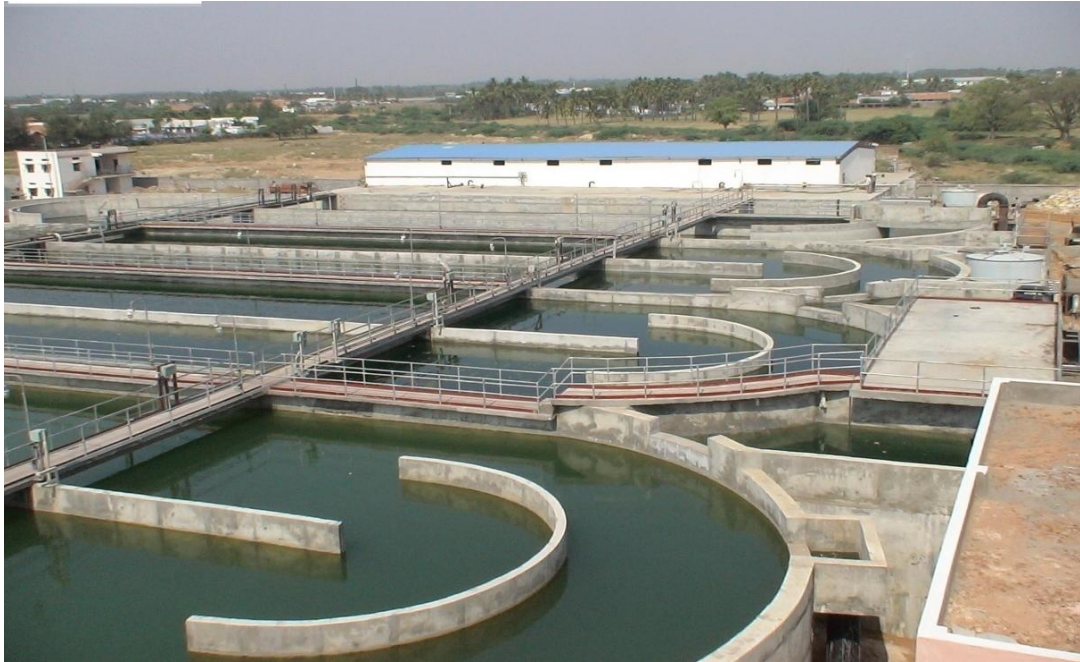
Biological Treatment Unit in Common Effluent Treatment Plant
