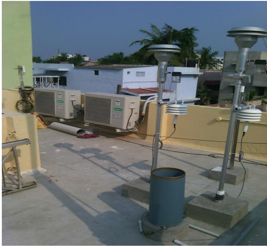
Continuous Air Monitoring Station At Perungudi
